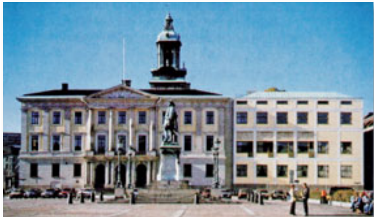
Abb. 6: Göteborg – Rathausbau, Arch. Gunnar Asplund, 1932
